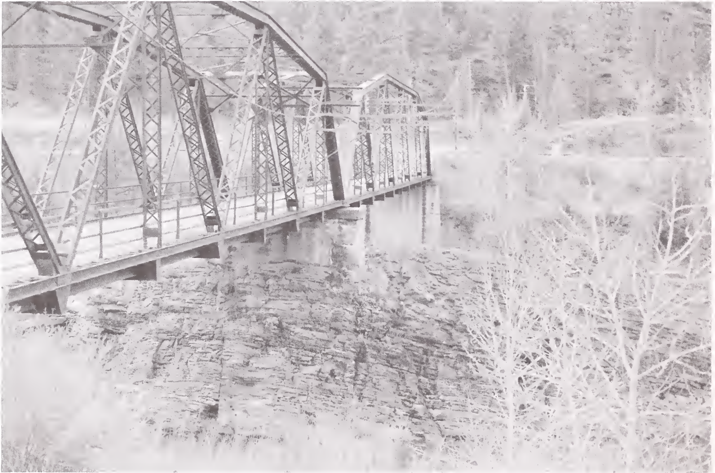
The Natural Pier Bridge in Mineral County.
